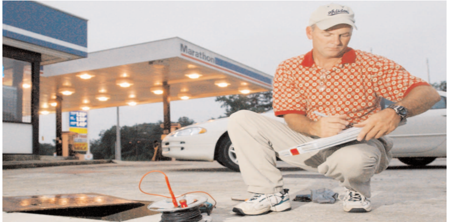
The well-traveled Harry Little captures cathodic protection data from an underground storage tank in Macon, Ga. (Photo by Woody Marshall)
