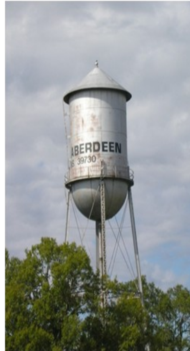
Steel is strong and durable. This steel water storage tank in Aberdeen, Mississippi, has been in continuous use for more than 100 years. STI/SPFA's Century Club recognizes many tanks like this throughout the US.
