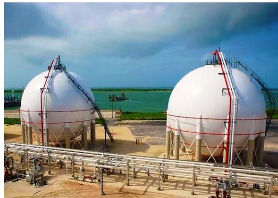
The Scope of Work for the spheres included the design and construction of the foundations, as well as the design and installation of the support columns including their fire proofing, multi ring deluge fire protection spray system, system piping from the sphere top to the ground, a galvanized stairway and field paint of the finished spheres and piping.
