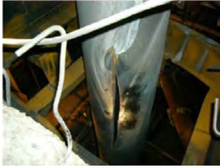
A steamline split recently in a 300MW unit at the Datong Power Station Unit 2 in China.
