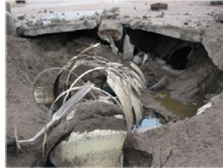
The lightning had entered through a fax/phone line in the facility building, causing little damage there. However, the current traveled to the underground FRP diesel and gasoline tanks, causing an explosion that leaked 625-700 gallons of fuel to the ground water, according to the report.
