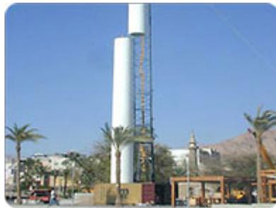
The largest free-standing flagpole in the world at 425 feet (129.5 meters) does its duty in Aqaba, Jordan. Made with A36 carbon steel, the 11-piece, urethane-coated pole was subjected to wind-tunnel and vortex studies to ensure that it could handle environmental conditions without external support. A 1,200-ton crane was used to erect the flagpole on site.
