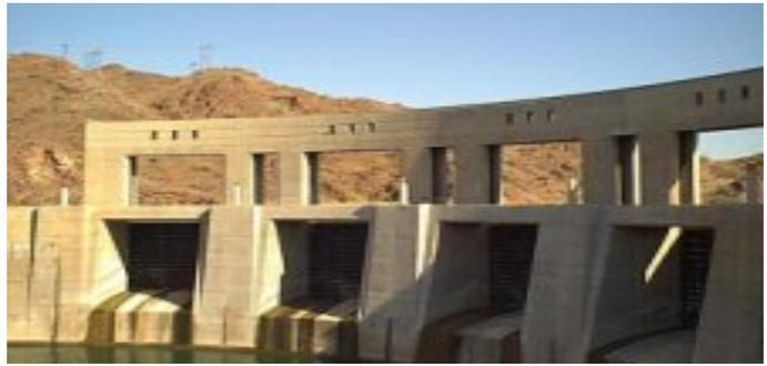
Approximately 73 percent of its structural height of 320 feet (97.5 meters) is below the original riverbed. Men and machines excavated 235 feet (71.6 meters) into the bed of the Colorado River before concrete was poured for the dam's foundation.
