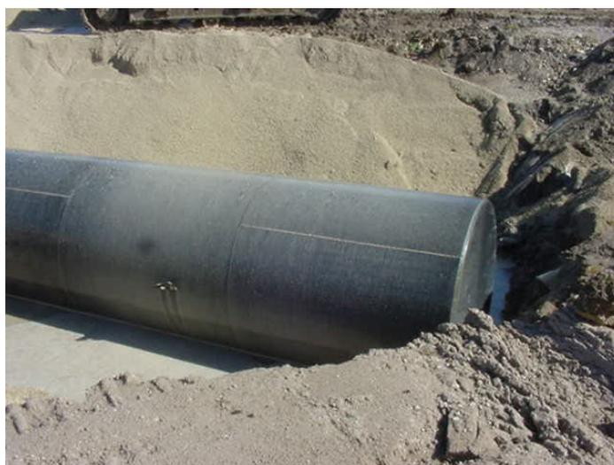
The steel tank shown above was tested to -15 psi—that's 30 times UL's standard for safety. Steel tanks are designed for negative pressures up to -0.5 psi.
