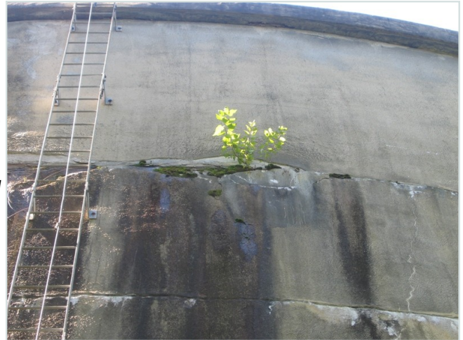
Many states require water storage tanks to be impervious. However, AWWA standards for concrete tanks have an allowable leakage rate as constructed. That means tank construction specifications must contain special instructions to be in compliance with those state regulations.
